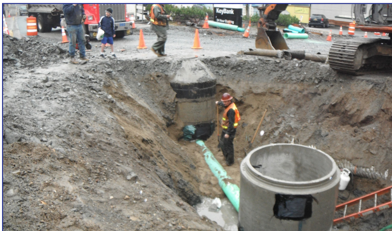
Crews install the sanitary sewer system along Main Street last summer. The large concrete structures will house the man holes that provide maintenance crews access for maintenance and repairs.
