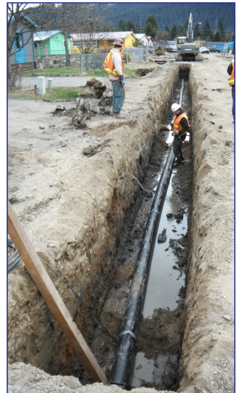
Crews install a new 8-inch water main in Eagles Edge Subdivision this spring.
