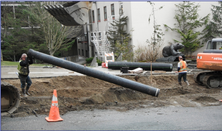
Water and sewer lines are usually located under roadways, so repairs and replacement are often done at the same time as road construction so that the road does not have to be torn up and repaved later. Here crews build a new water main under Juneau's Main Street last summer.
